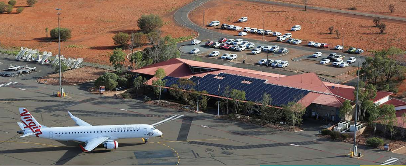
Solar panels on Ayers Rock Airport. Photo: Voyages.
