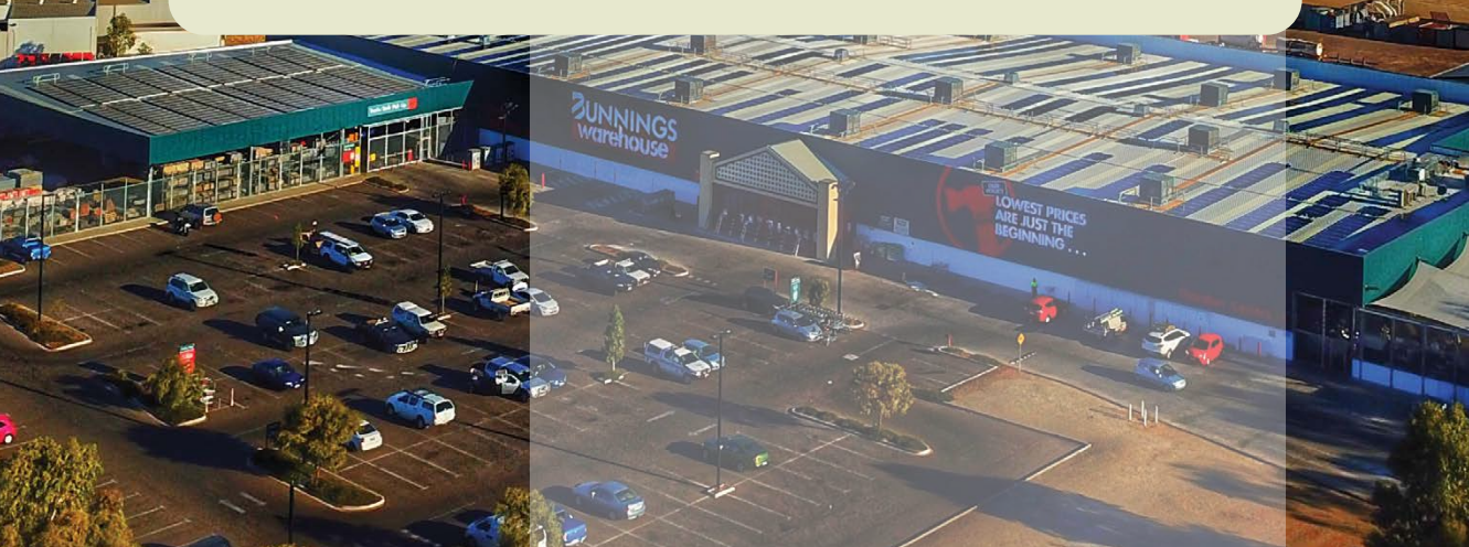
Rooftop solar at Bunnings Warehouse, Alice Springs. Photo: Bunnings Group Limited.
