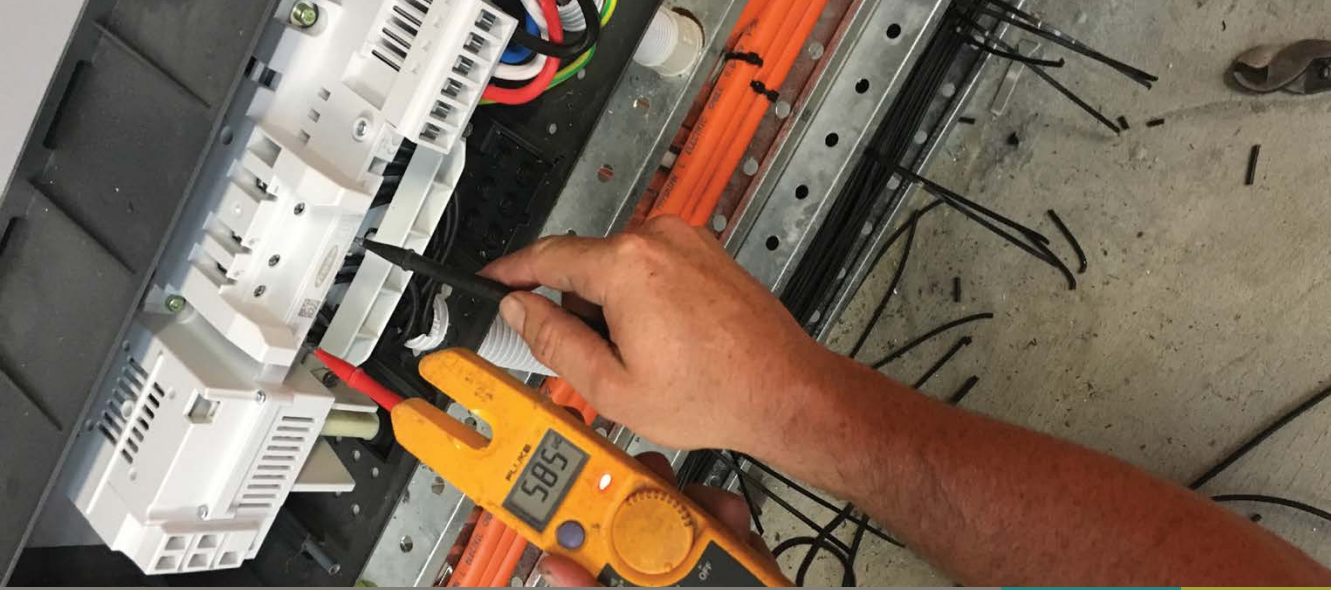
Inspecting a solar PV installation. Photo: ECG Electrical.
