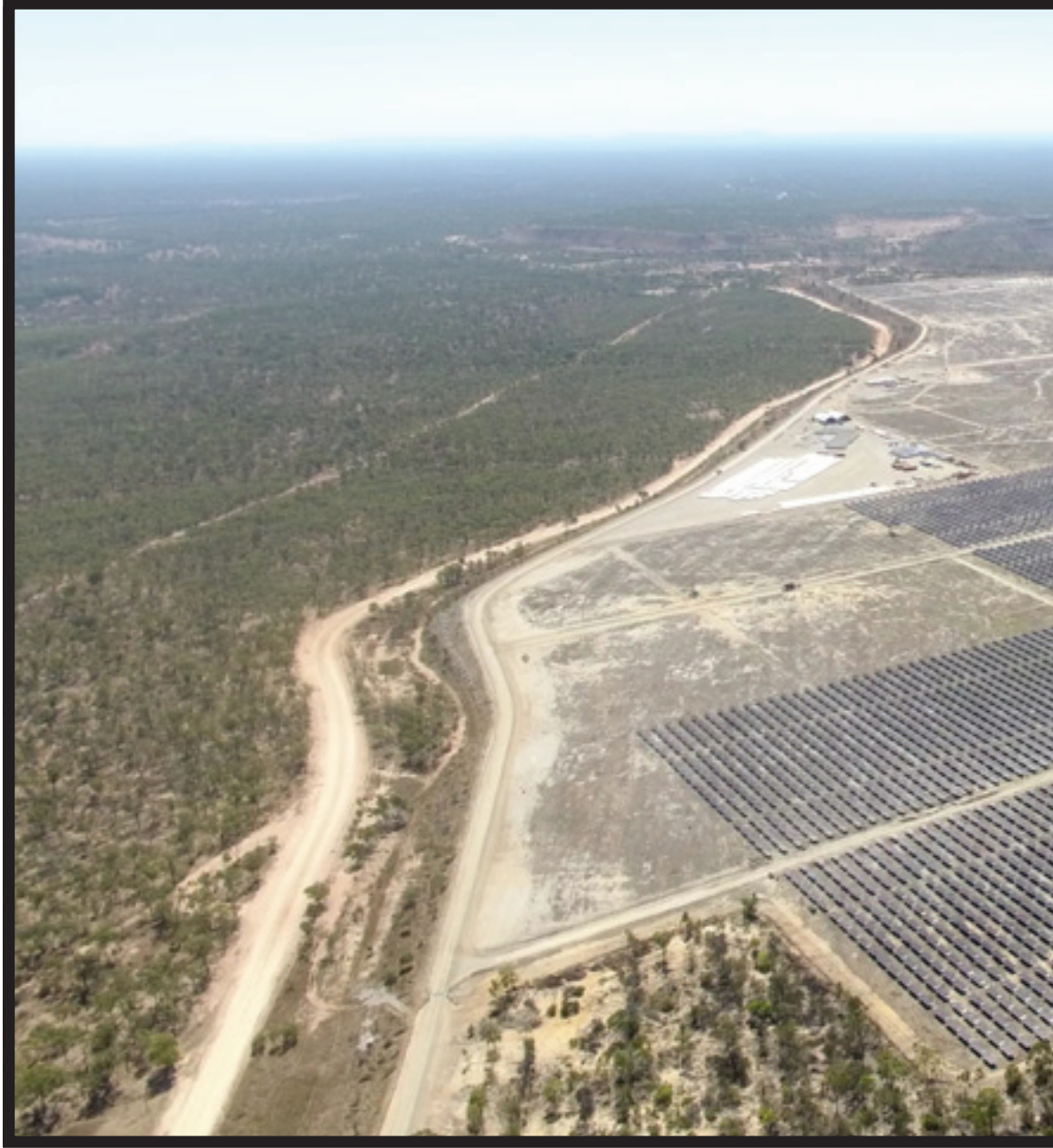
Photo: Kidston Solar Project, Genex Power, Qld
