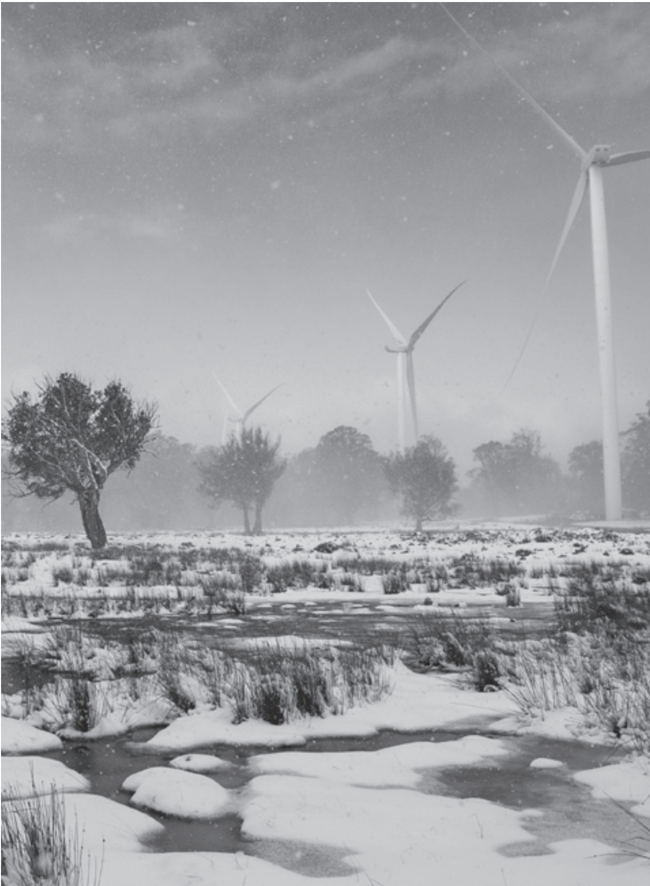
Photo: Cattle Hill Wind Farm, Lake Echo, Tasmania
